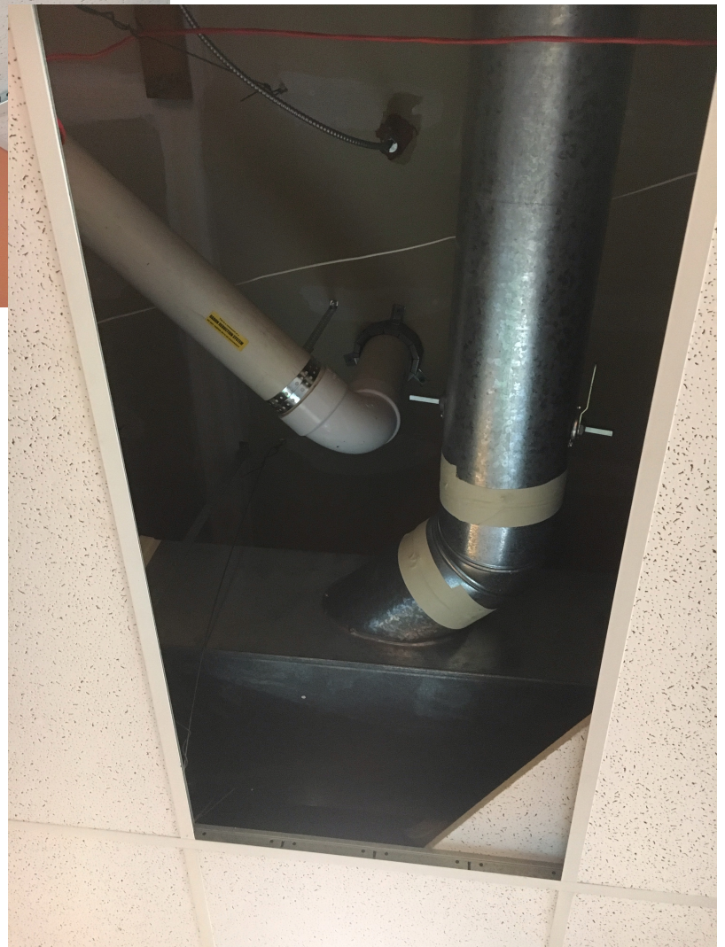
Vent piping continues through the drop ceiling of the media center to the fan location on the roof.
