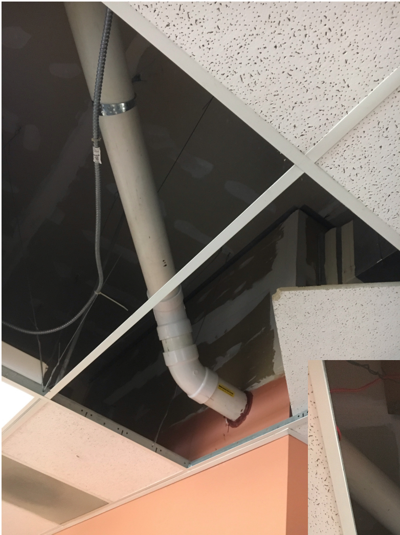
Vent piping coming from the suction point location in the mechanical storage room.
